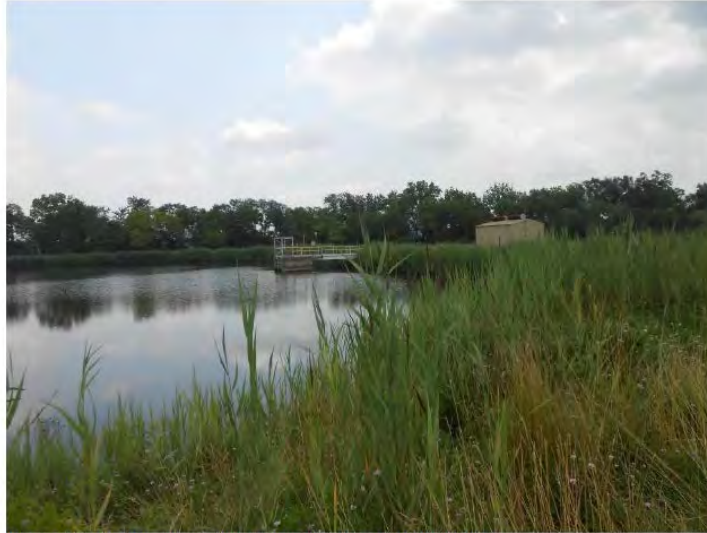
Photo 29 – Outlet structure between basin and polishing pond.
