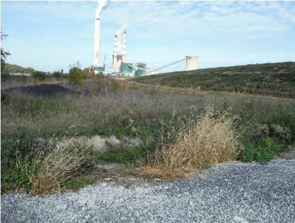
Photo 2 – West edge of Active Cells A and B. The berm to the left of the photo separates active Cells A-B from Cells C-D, which have not yet been constructed. The berm overlies the two 48-inch pipes that divert an existing stream through the Landfill footprint.
