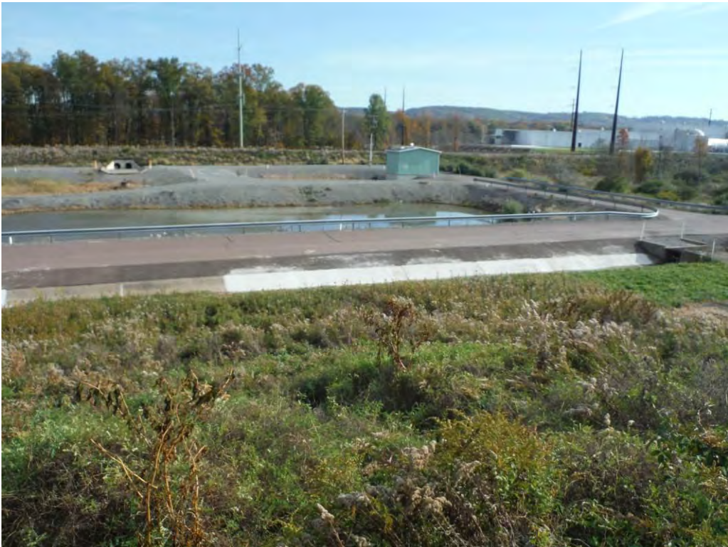
Photo 15 – Leachate runoff basin, looking south.
