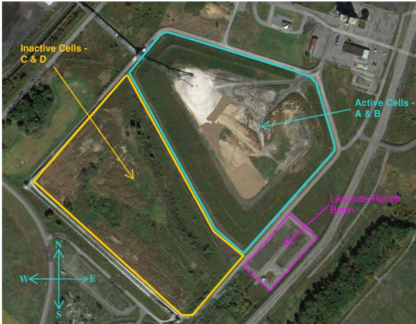
Photo 1 - Aerial view of Montour Ash Area No. 3. Cells A and B, which are actively being filled, can be seen in the center. Construction of Cells C and D has not yet started.
