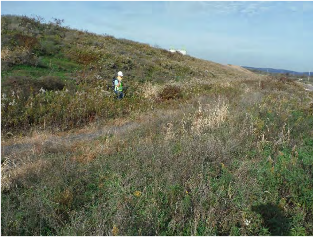
Photo 4 – East side of Cells A and B, showing heavy vegetation.
