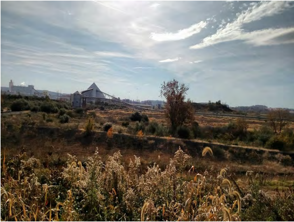
Photo 14 – Inactive Cells C and D, looking west.
