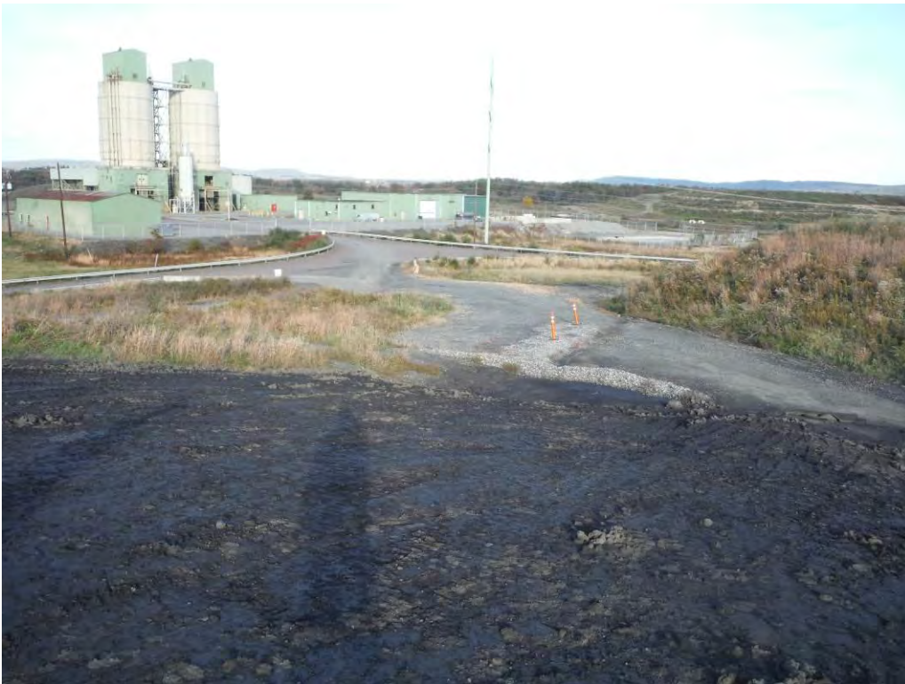
Photo 9 – Access road, looking east. Erosion control measures did not appear to be capable of preventing stormwater runoff from flowing down the road and out of the Landfill.
