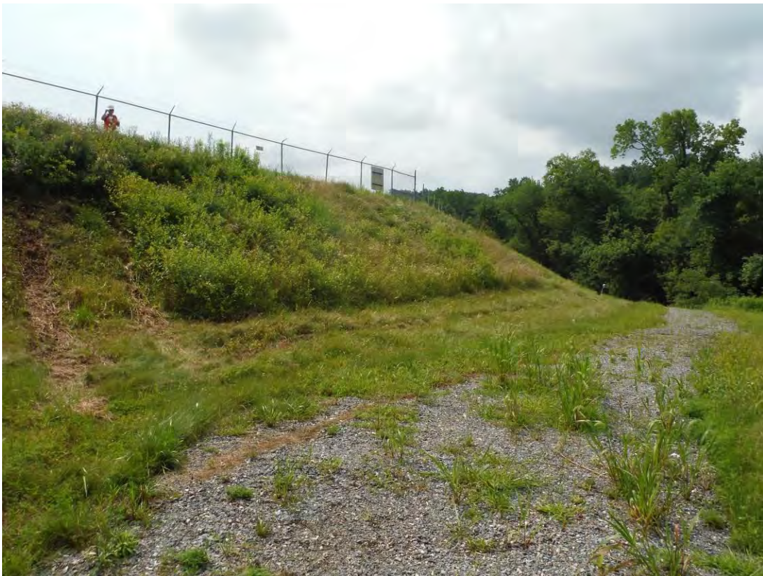
Photo 11 – Downstream slope of the north embankment near the northwest corner, showing a section of the slope where vegetation was not recently cut.
