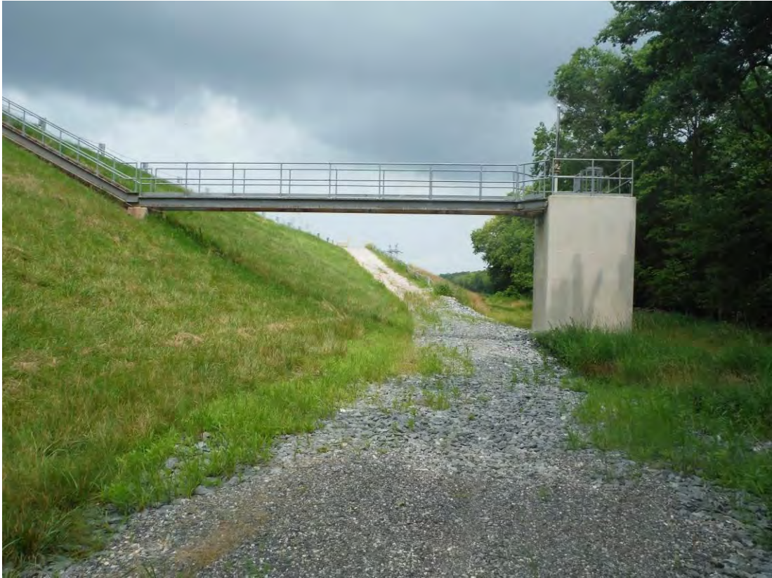
Photo 12 – South embankment at the polishing pond discharge regulating structure, looking north.
