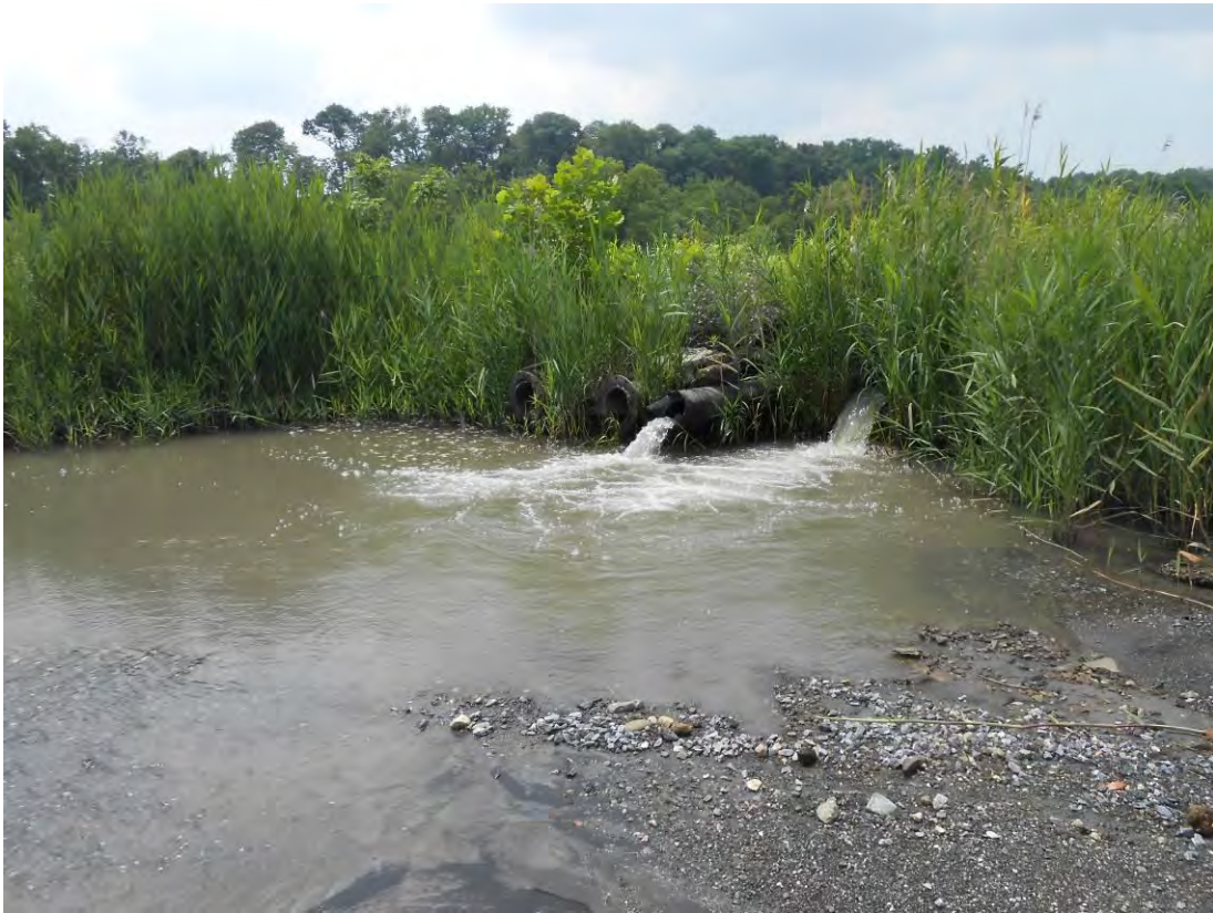
Photo 28 – Former ash slurry discharge location near the northwest corner of the basin. The discharge pipes in the center of the photo are still being used to discharge process water.
