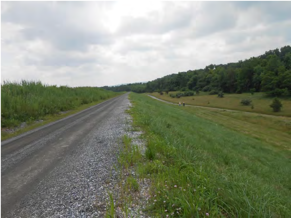
Photo 26 – Crest of the west embankment, looking south from bend.
