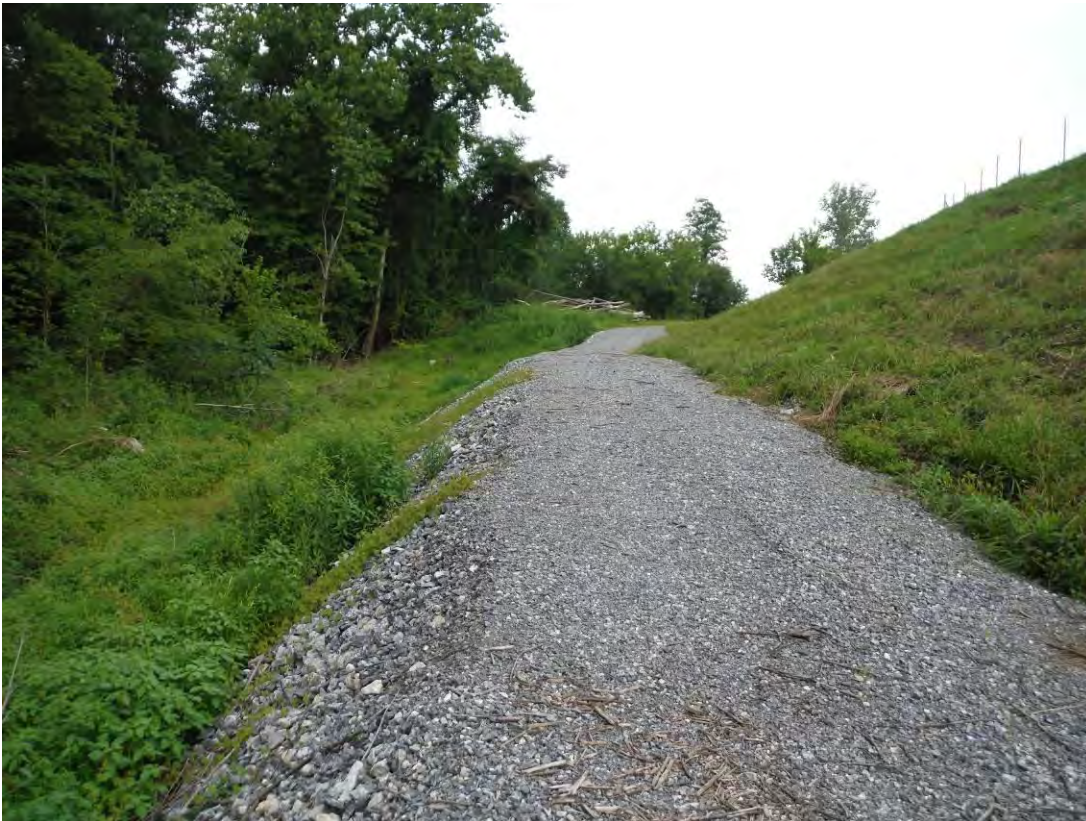
Photo 25 – Area of historic slough at the north end of the west embankment which was recently repaired. An access road with a stone berm was recently constructed. Note vegetation at toe.
