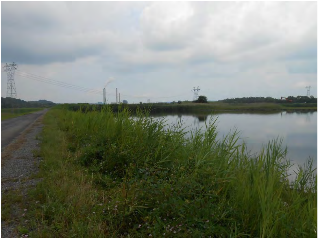
Photo 27 – Vegetation along the upstream slope of the west embankment.
