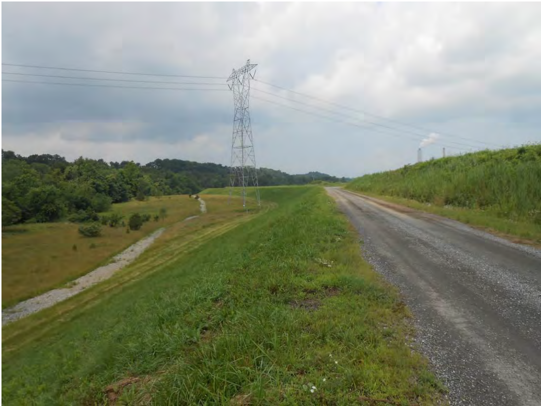
Photo 18 – Downstream slope of the west embankment, looking north from Station 9+00W.
