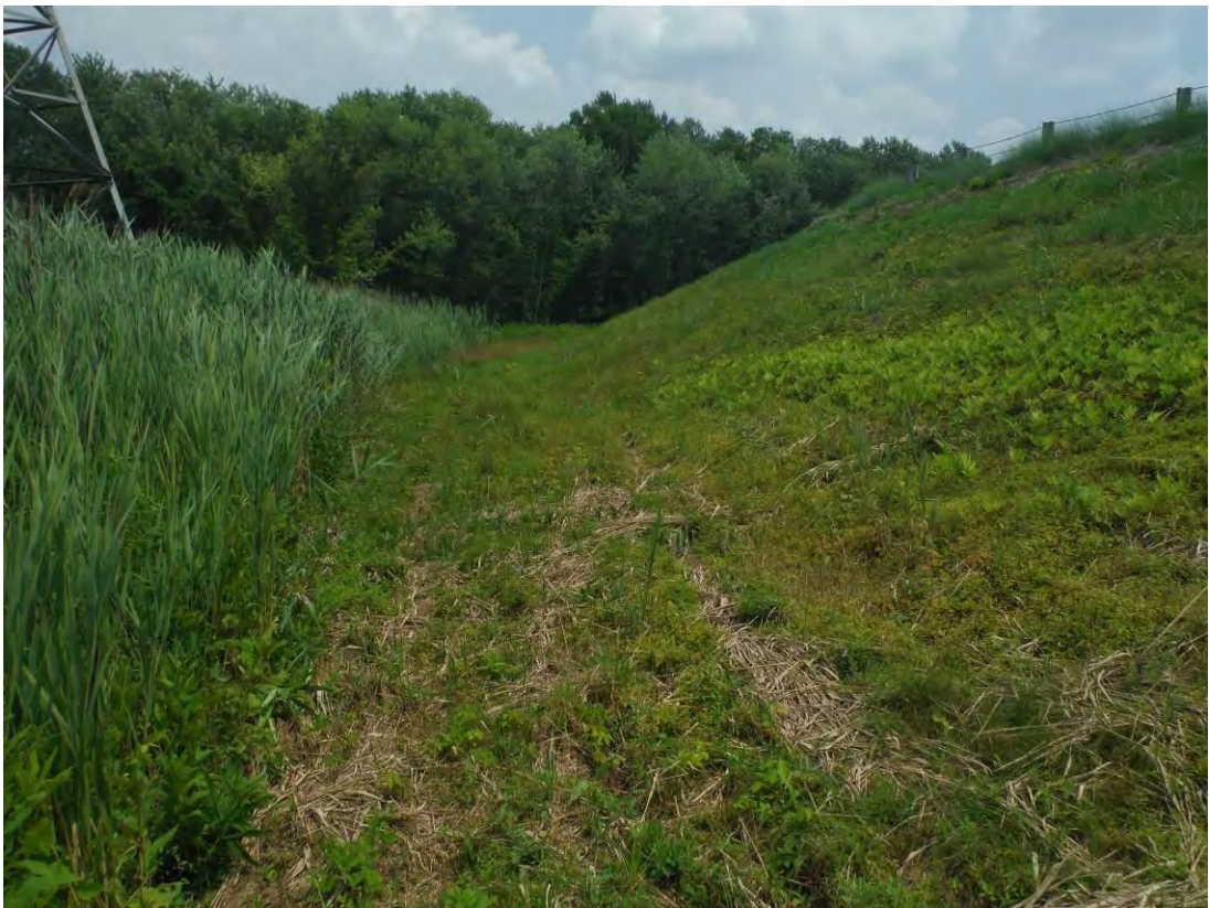
Photo 9 – Downstream slope of the embankment at the northeast corner, looking east.
