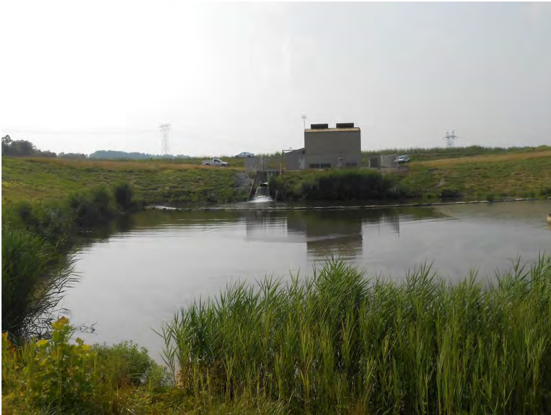
Photo 30 – Median dike, metering station, and discharge structure to the polishing pond, looking north.
