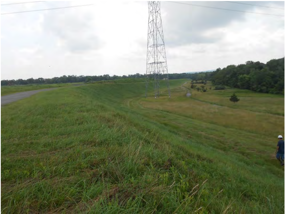
Photo 19 – Downstream slope of west embankment, looking south.
