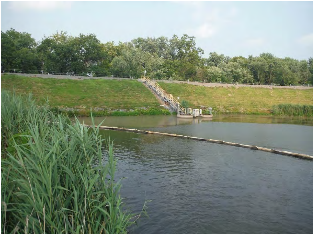
Photo 33 – Outlet structure in the polishing pond.
