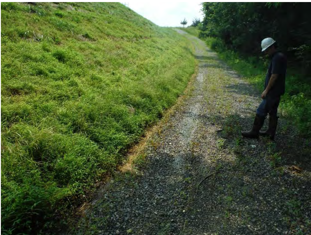
Photo 21 – Wet area with standing water at the north end of the west embankment in a previously disturbed area that had been restored.
