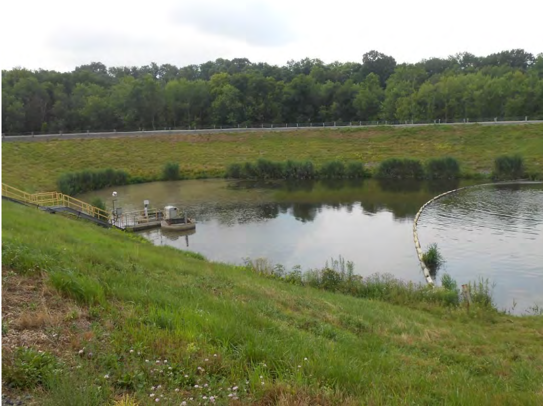
Photo 15 – Interior slope of the polishing pond, looking south.
