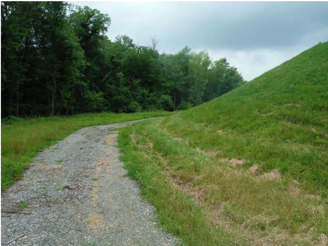
Photo 13 – Downstream slope of the south embankment looking west.
