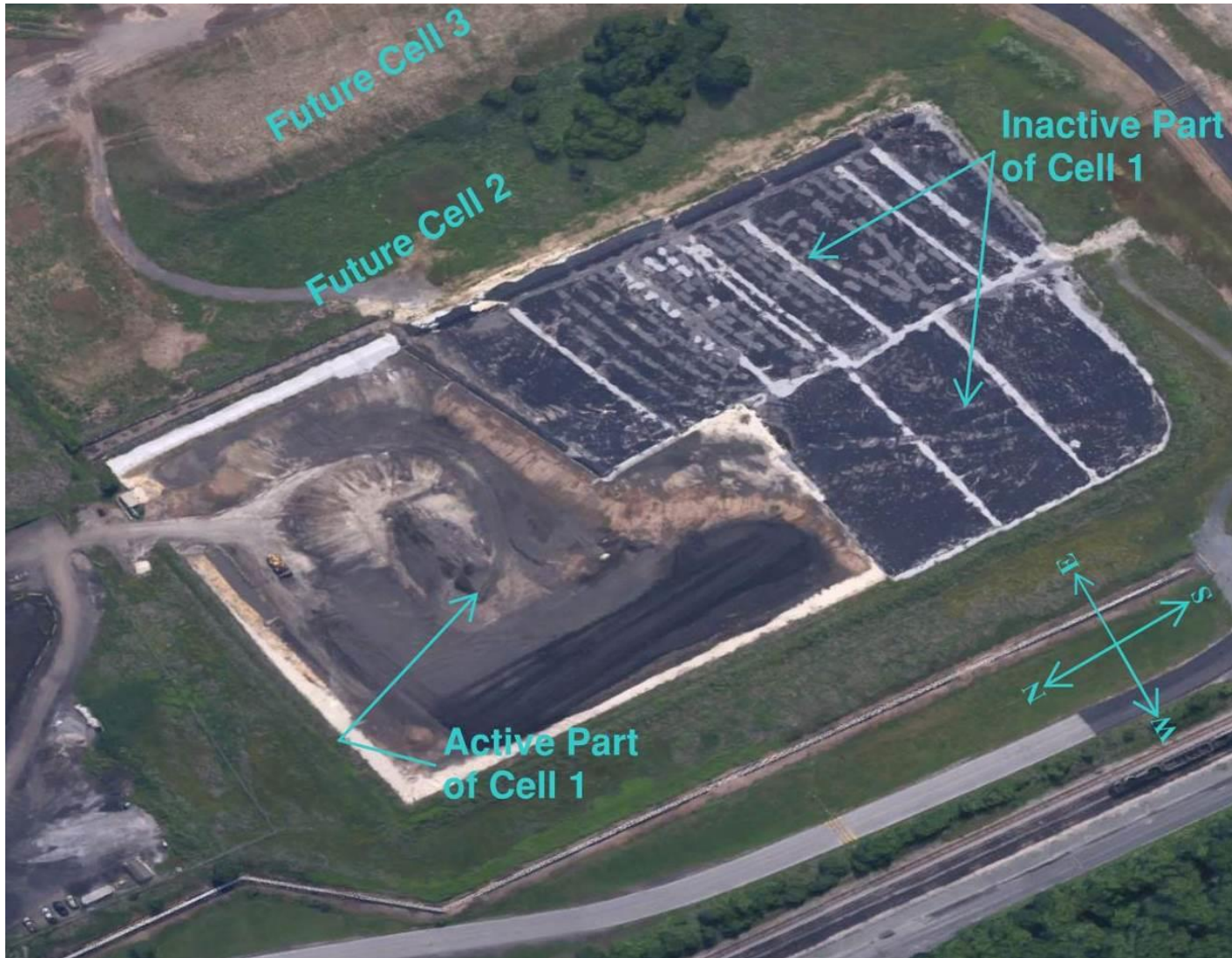
Photo 1 - Aerial view of Brunner Island Ash Area No. 8. The active part of Cell 1 is seen to the left (north). The right (southern) part of Cell 1 has had the liner system installed, but has not been filled. Temporary plastic tarps can be seen covering the liner system over the inactive part of Cell 1. Construction of Cells 2 and 3 has not yet started.
