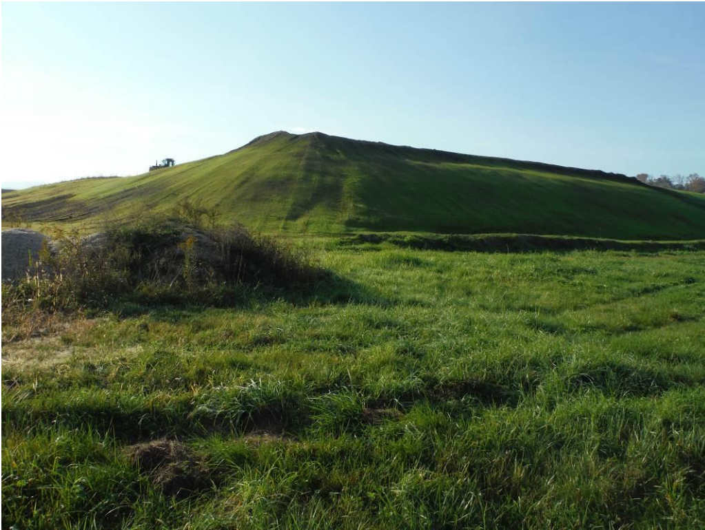
Photo 2 – North and east slopes of the active part of Cell 1. The final build out of the slopes has not taken place and the vegetative cover is temporary, providing erosion and dust control.
