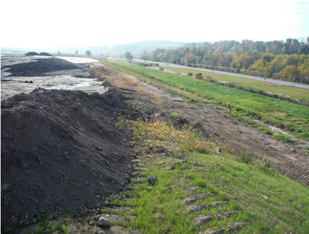
Photo 15 – West edge of Cell 1 showing containment measures under construction. .
