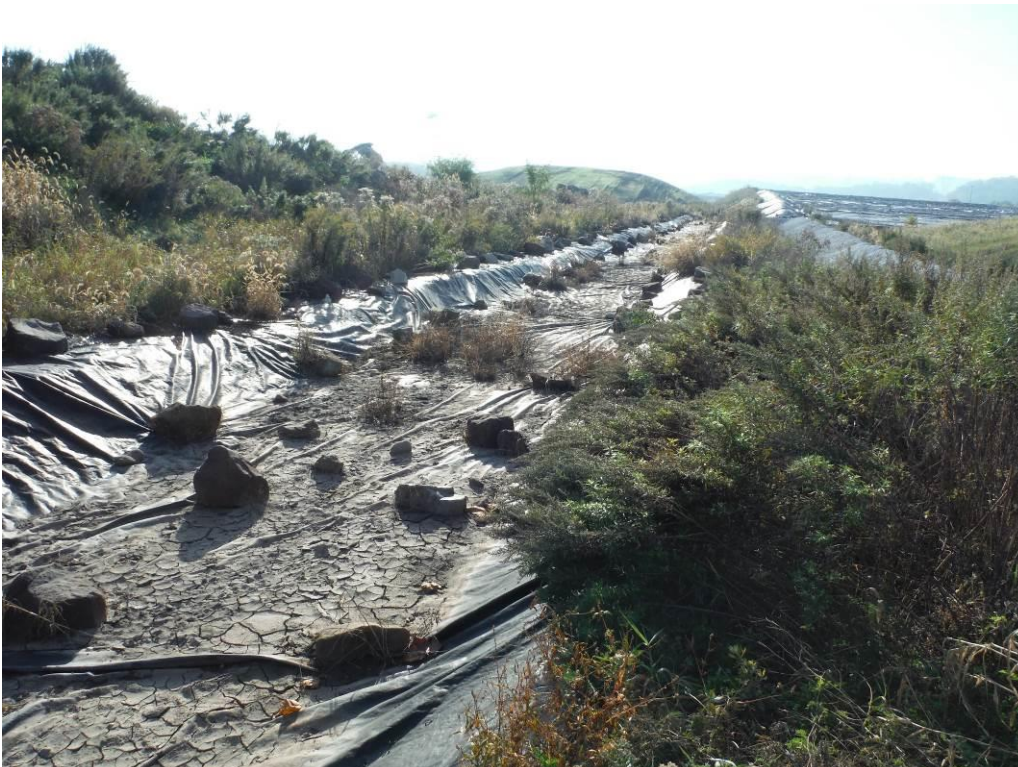
Photo 7 – Clean water discharge channel draining the unfilled part of Cell 1. This discharges to a ditch leading to the Susquehanna River.
