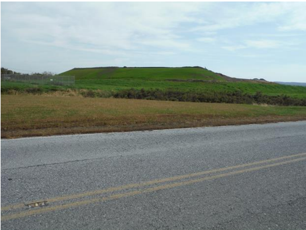
Photo 3 - North and west slopes of the active part of Cell 1.
