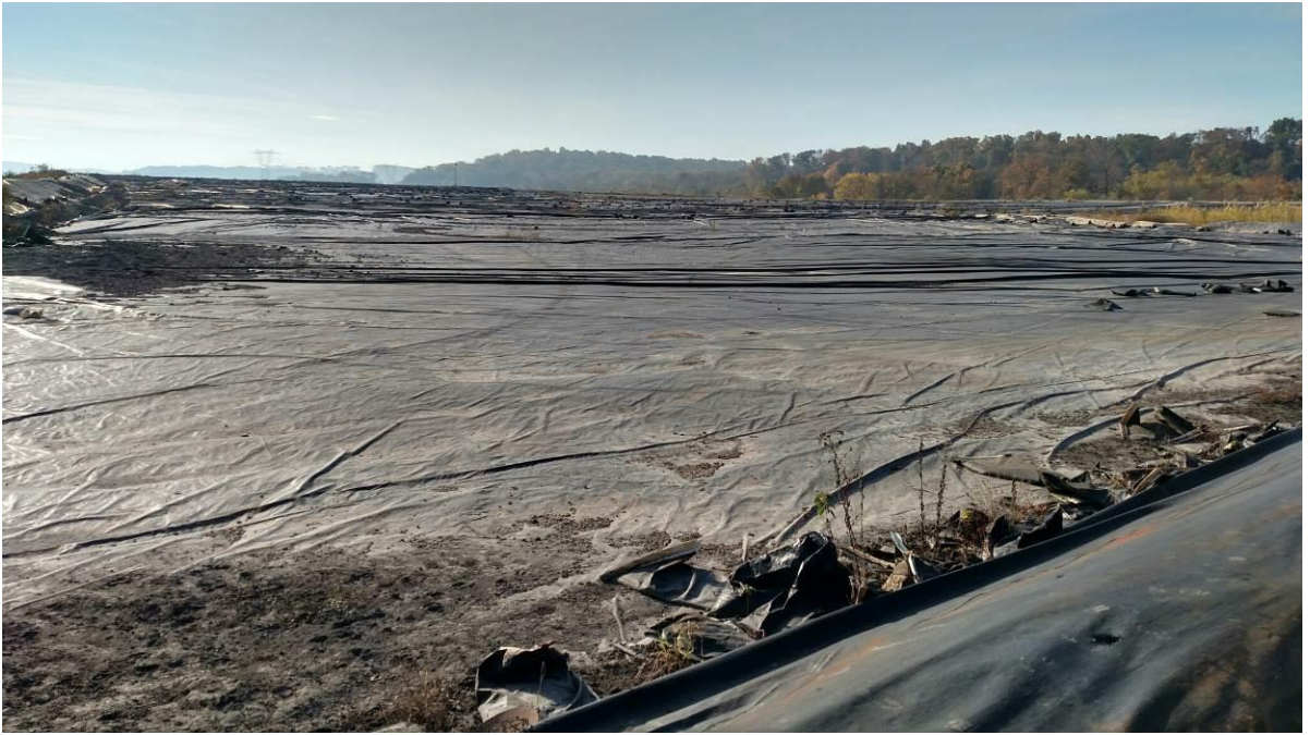
Photo 4 – Unfilled (inactive) section of Cell 1. Note the temporary plastic tarps covering the liner system.
