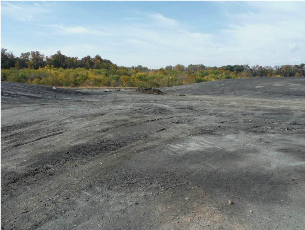
Photo 14 – Landfill surface, showing grading and finishing of the working surface. A recently dumped load can be seen in the photo center.
