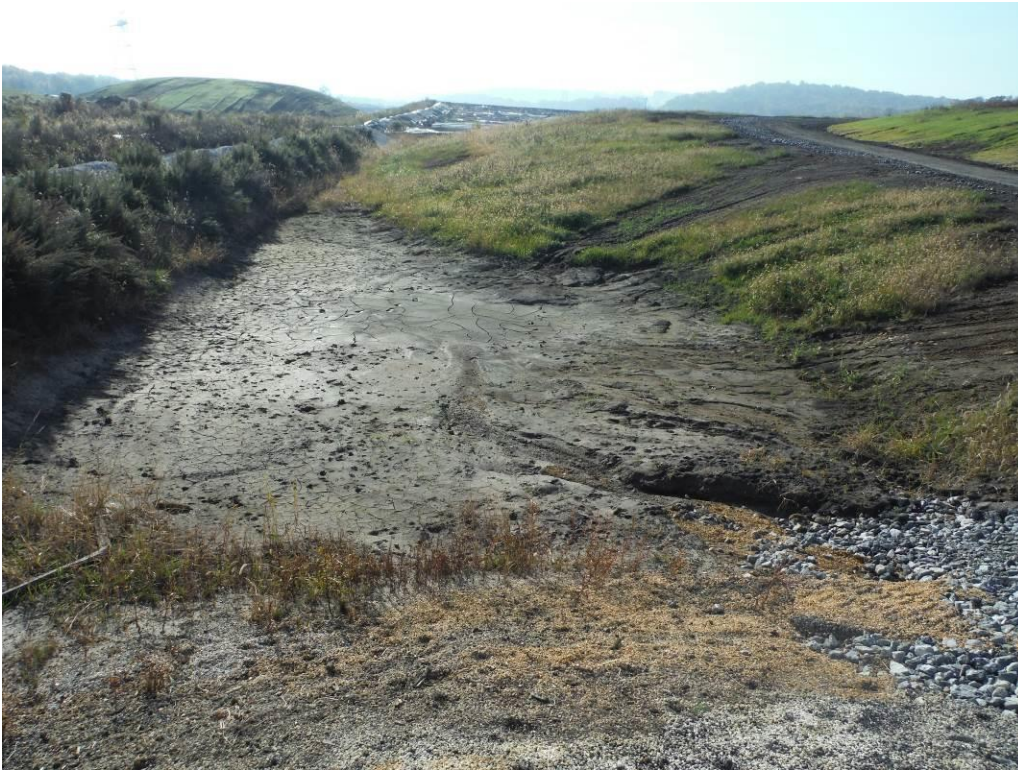
Photo 6 – Ditch separating Cell 1 from future Cell 2. The swale surrounding the active part of Cell 1 drains to the temporary stormwater detention basin shown in the foreground. Captured stormwater percolates to the sump and is pumped to the Plant Flue Gas Desulfurization (FGD) waste water treatment plant. The clean water channel shown in Photo 7 is to the left.
