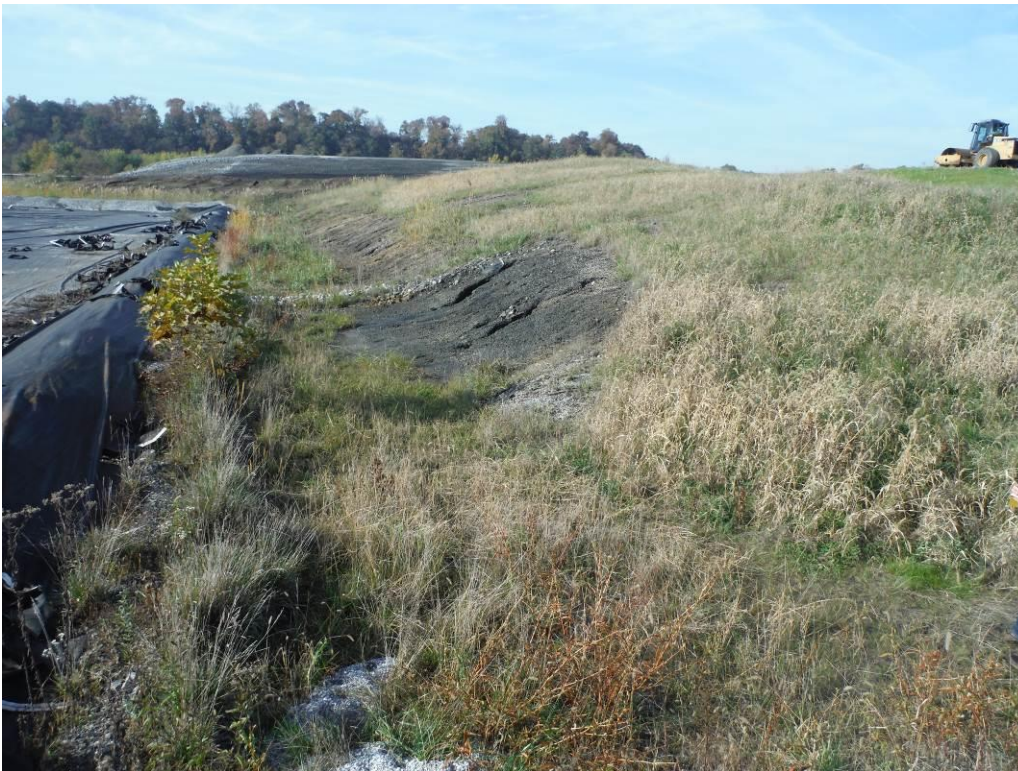
Photo 13 – South edge of the active part of Cell 1, showing temporary vegetation used for erosion control and a locally steep area subject to erosion.
